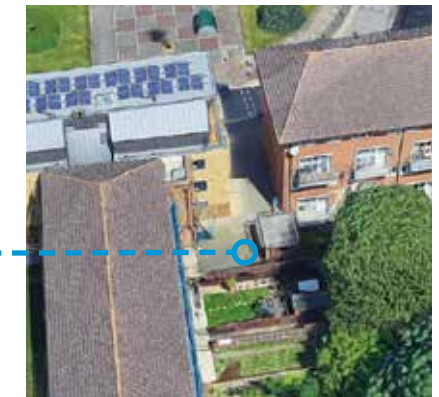
4) Between Glebe House and Cornick House
