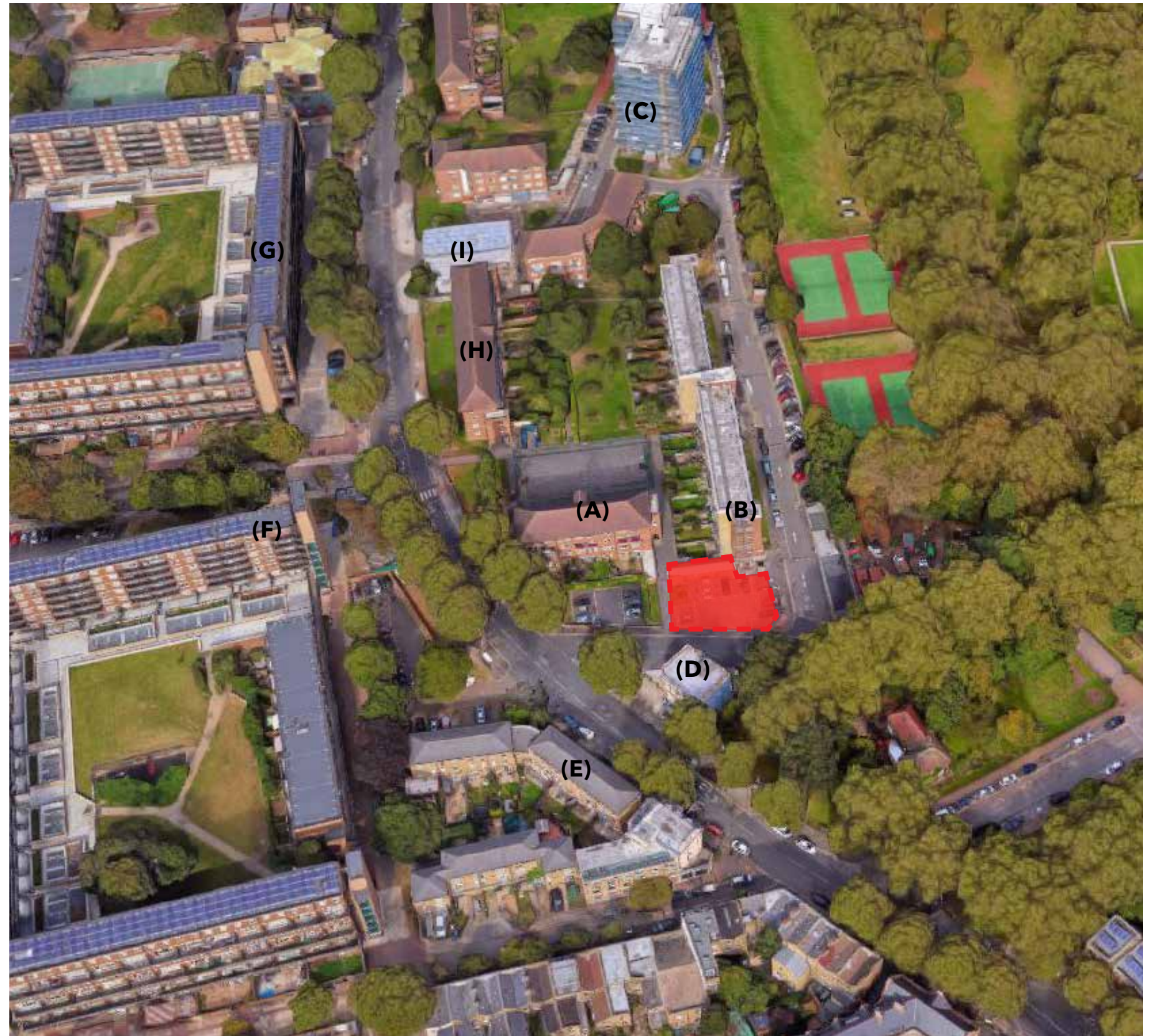
Aerial view with storey heights
