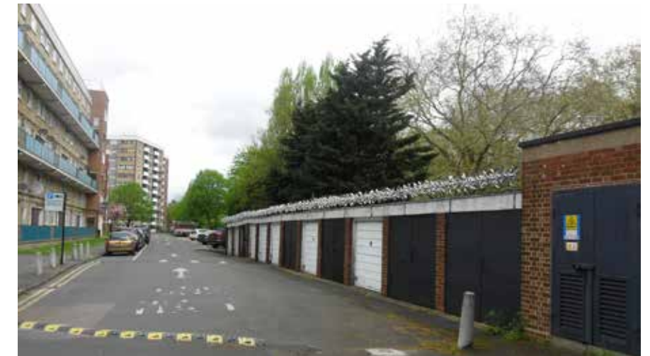
2. View of the existing garages to the east of Matson House
